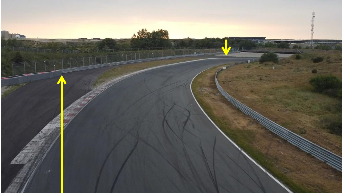
Asfalt run off area
